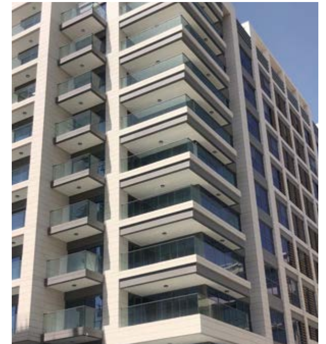
DHAFRA PROJECT - ABU DHABI RESIDENTIAL BUILDING
